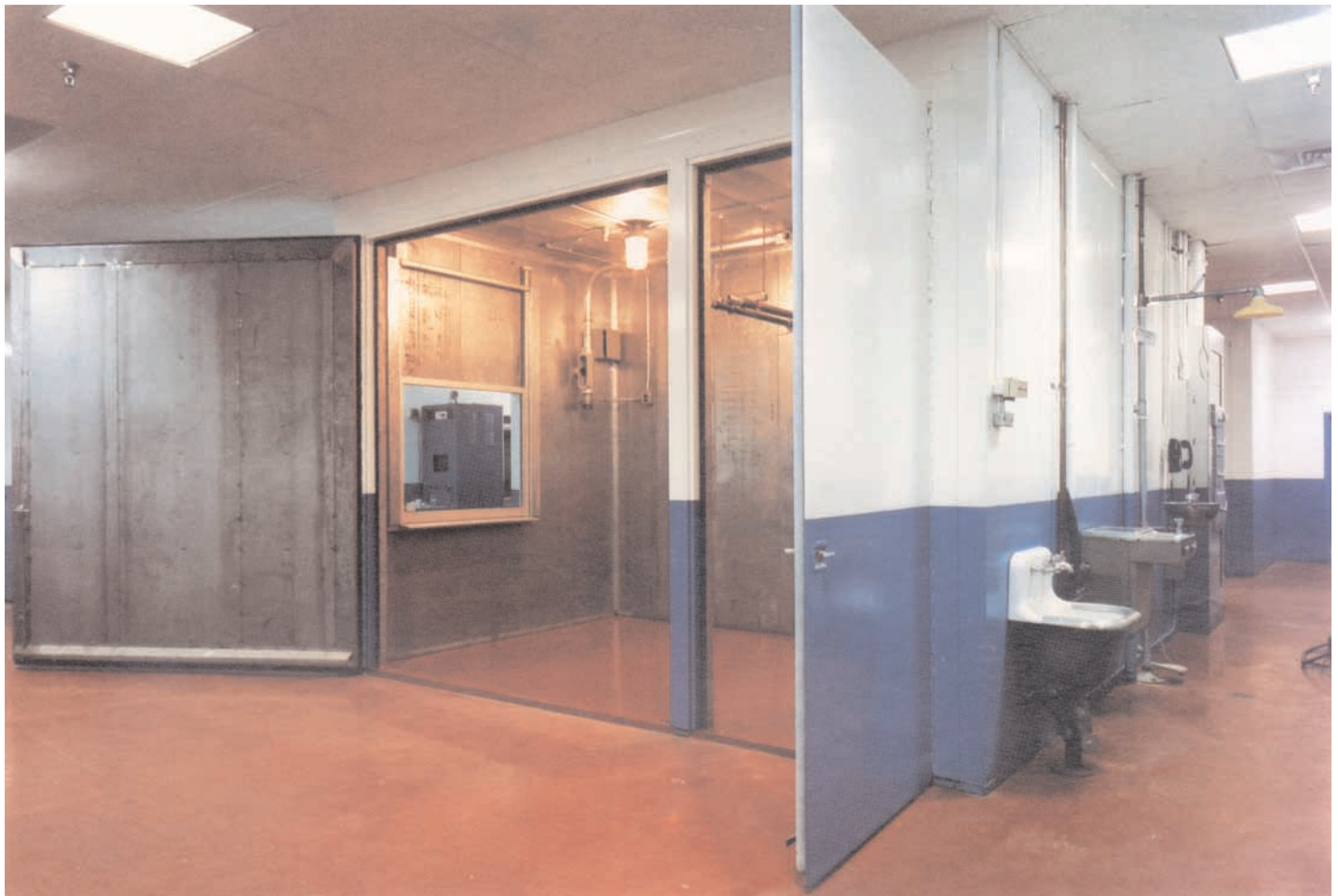
Careful door construction and assembly allow these 9-foot by 10-foot doors to be opened and closed by one operator. These doors have what I call a Cadillac action, said Al Roberts, Vickers Plant Engineer.
