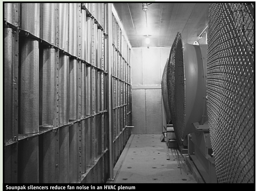
Sounpak silencers reduce fan noise in an HVAC plenum
