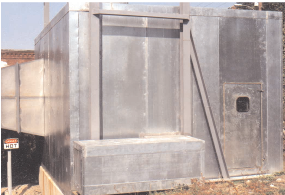
The 12-foot-high SOUNDSCREEN enclosure came supplied with access doors and a ventilation system to keep temperatures in the housing down.
